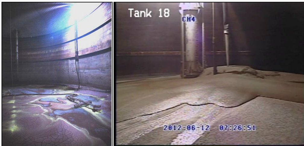
Figure 5: SRS Tank 18 Being Filled with Cementitious Material
