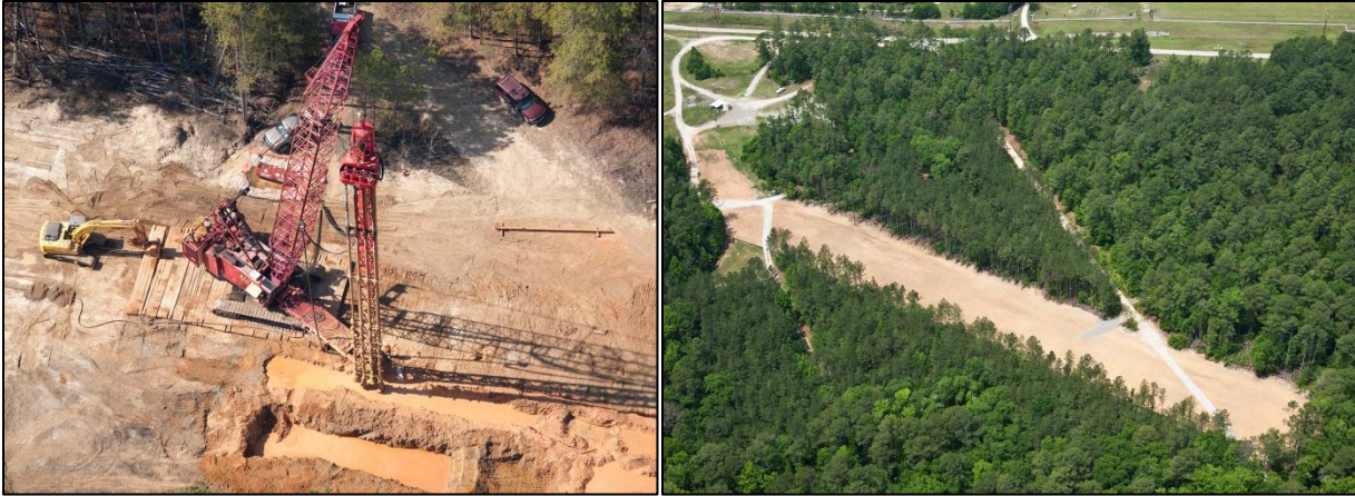
Figure 7: F-Area Seepage Basin Grout Wall During (Left) and After (Right) Installation at SRS.
